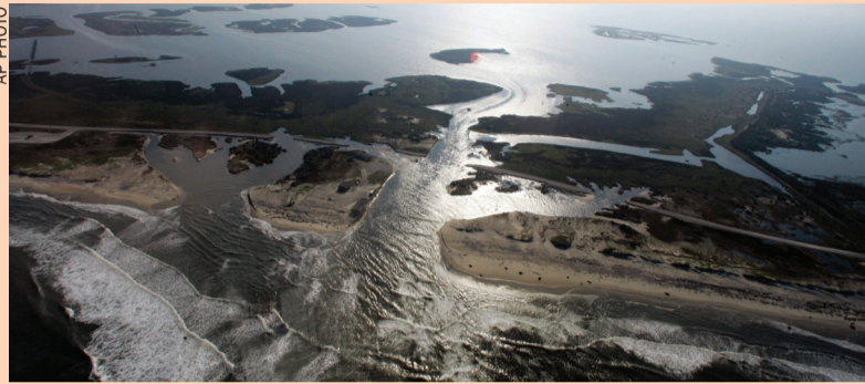
A flooded road on Hatteras Island, N.C., after Hurricane Irene swept through the area the previous day cutting the roadway in five locations
