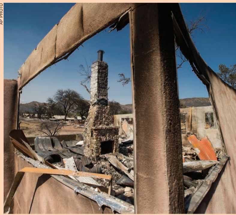
A chimney stands amid rubble at a house scorched by a wildfire in Phelan
