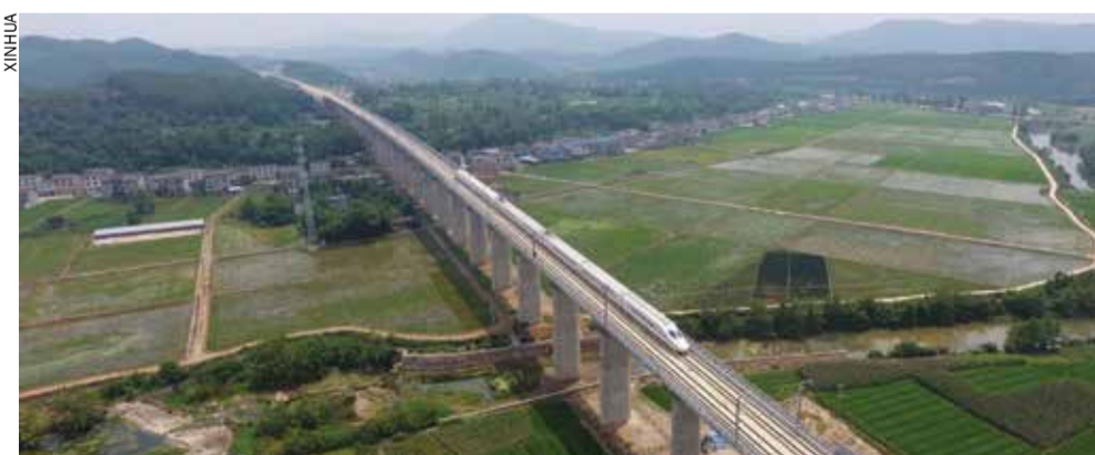
A train runs on Wangjiaba Bridge during a joint test of the Sichuan section of Xi'an-Chengdu Passenger Railway in Jiangyou. The first high-speed railway travelling through the Qinling Mountains with a projected speed of 250 kilometers per hour, started a joint test Monday in its Sichuan section
