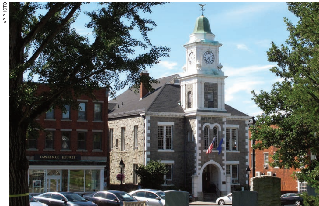
The Litchfield Judicial District Courthouse in Litchfield, Connecticut, which was closed on August 25 by the state authorities
