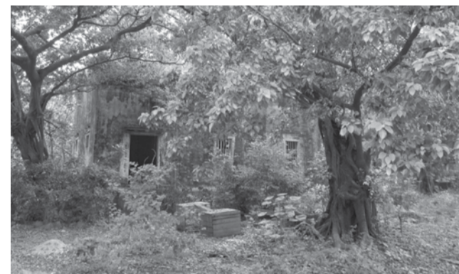
Inside the decrepit Iec Long Firecracker Factory
