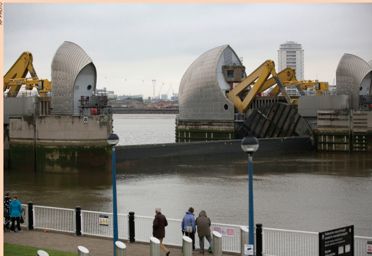
A sector gate on the Thames Barrier reopening for one of its monthly tests on the River Thames in east London
