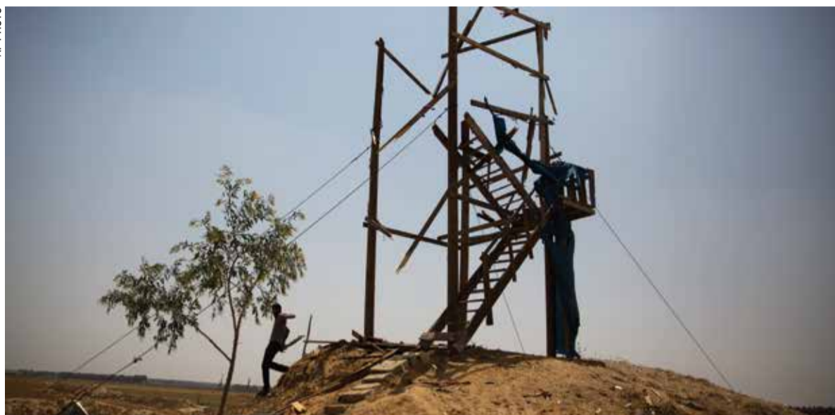
A Palestinian man inspects a military observation post that was hit by an Israeli tank shell in Khan Younis, southern Gaza Strip
