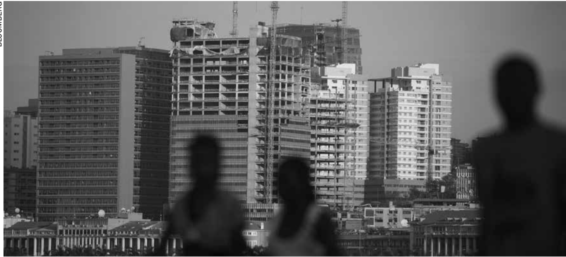
Construction cranes operate among new skyscrapers being built in the business district of Luanda
