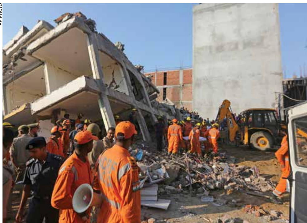
Rescue workers carry the body of a victim from the site of a collapsed building in Shahberi village, east of New Delhi, yesterday
