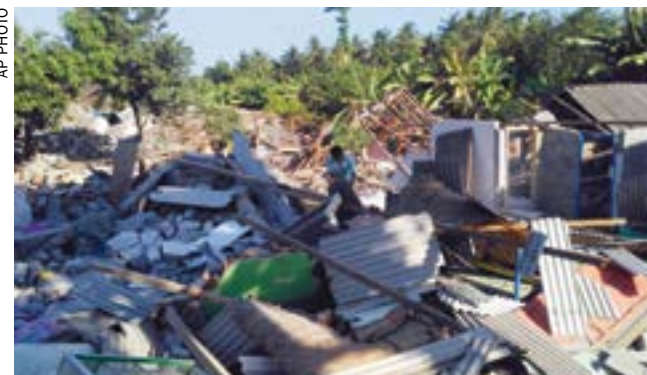
A man inspects destroyed homes following yesterday's earthquake on Lombok island
