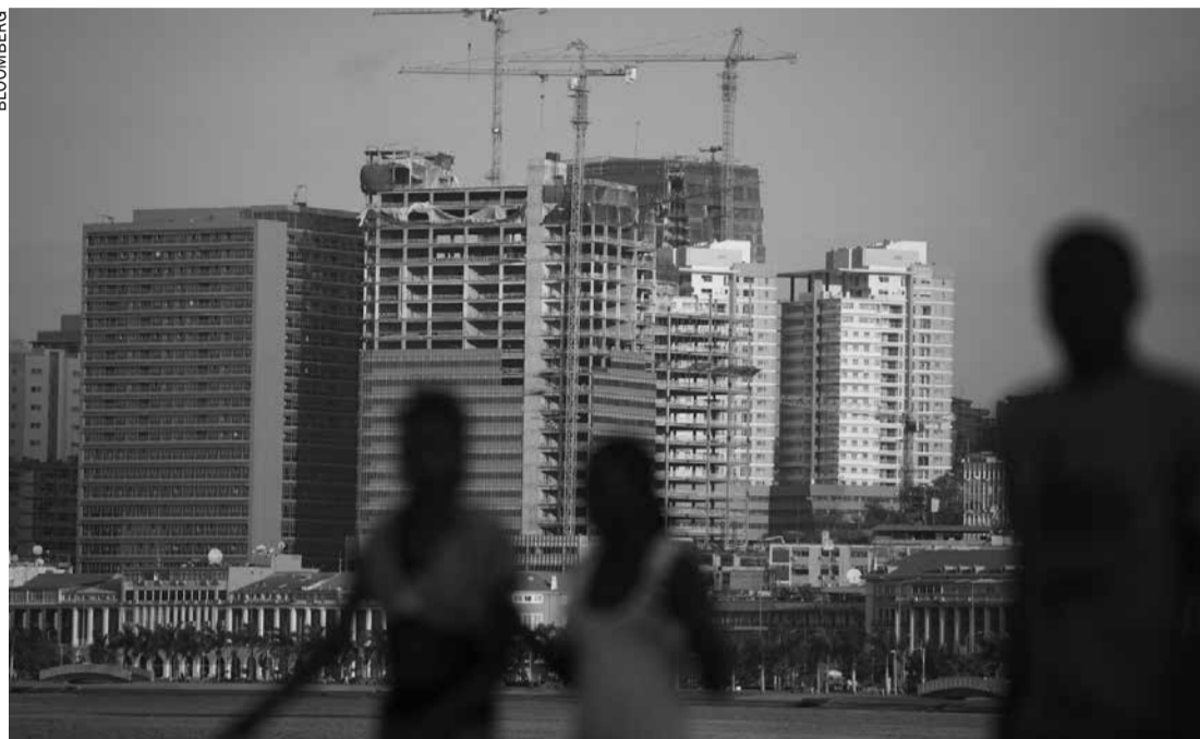
Construction cranes operate among new skyscrapers being built in Luanda
