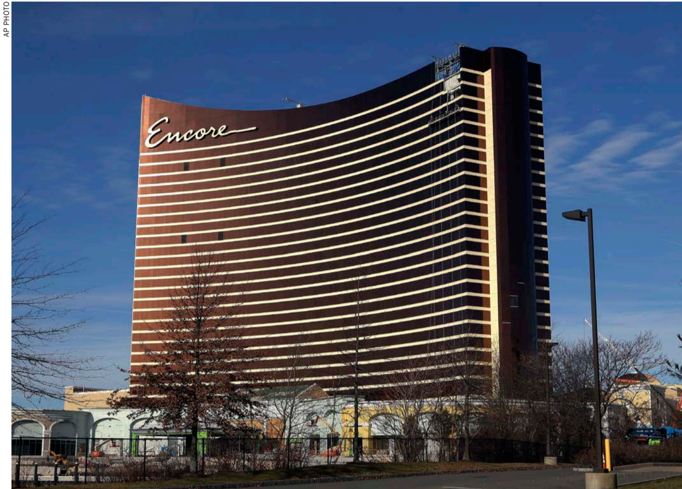
In this January 2 file photo, construction continues on the Encore Boston Harbor luxury resort and casino in Everett, Massachusetts
