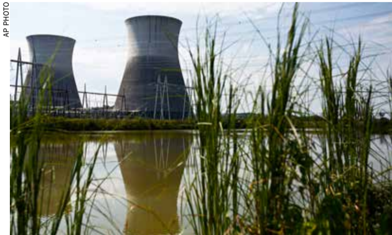
Two cooling towers can be seen outside of the Bellefonte Nuclear Plant, in Hollywood
