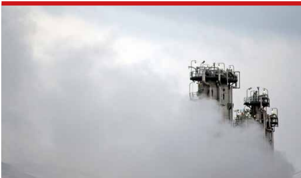
A part of Arak heavy water nuclear facilities, near the central city of Arak, 250km southwest of Tehran
