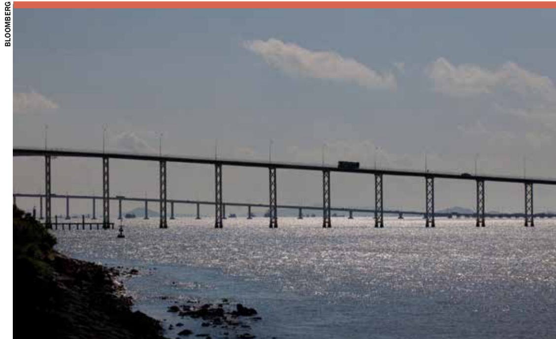
The Governor Nobre de Carvalho Bridge (foreground) and the Friendship Bridge link Taipa island to the Macau peninsula
