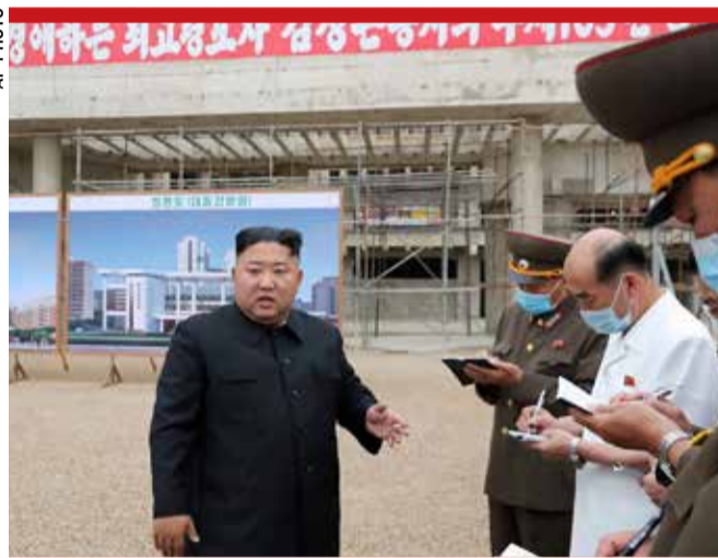
North Korean leader Kim Jong Un (center) visits a construction site of a hospital in Pyongyang
