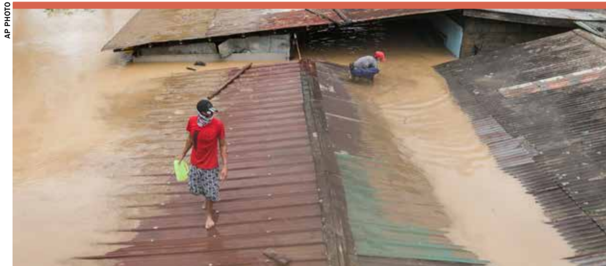
A man walks on top of a roof of a submerged house as floods inundate villages in Rizal province yesterday
