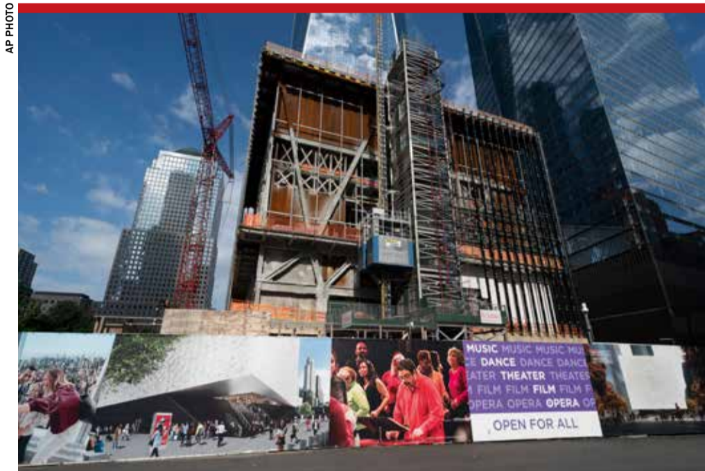
The Ronald O. Perelman Performing Arts Center is under construction
