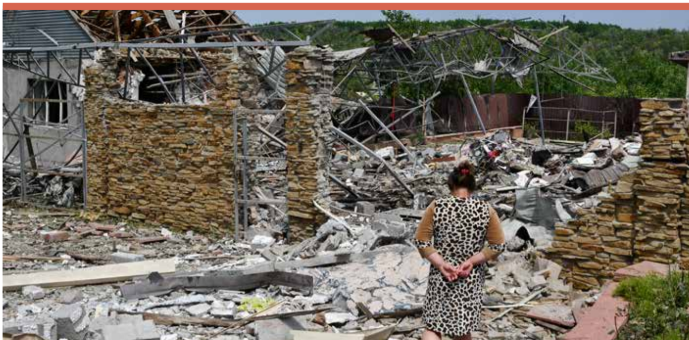
A building damaged by an overnight missile strike in Sloviansk
