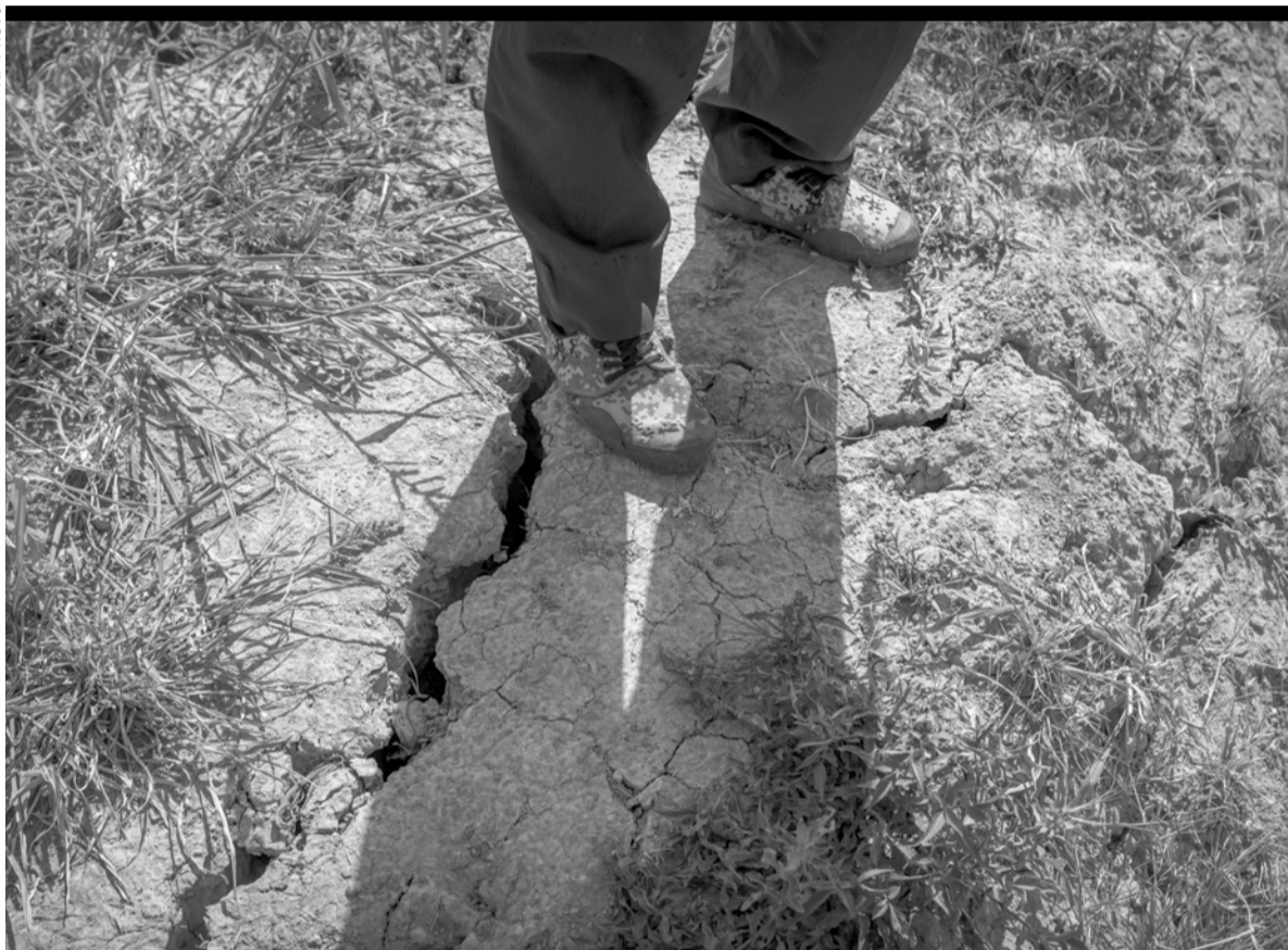
A farmer stands above a deep crack in the dried mud of an earthen embankment in his rice fields on the outskirts of Chongqing
