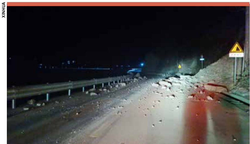
Fallen rocks after a landslide are seen on a road to Moxi Township in Garze Tibetan Autonomous Prefecture, southwest China's Sichuan Province early yesterday
