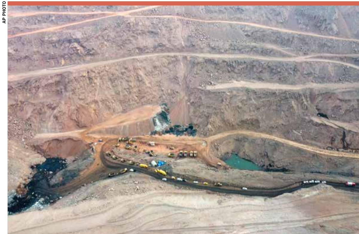
In this aerial photo, rescuers work at the site of a collapsed open pit coal mine in Alxa League in northern China's Inner Mongolia Autonomous Region, yesterday
