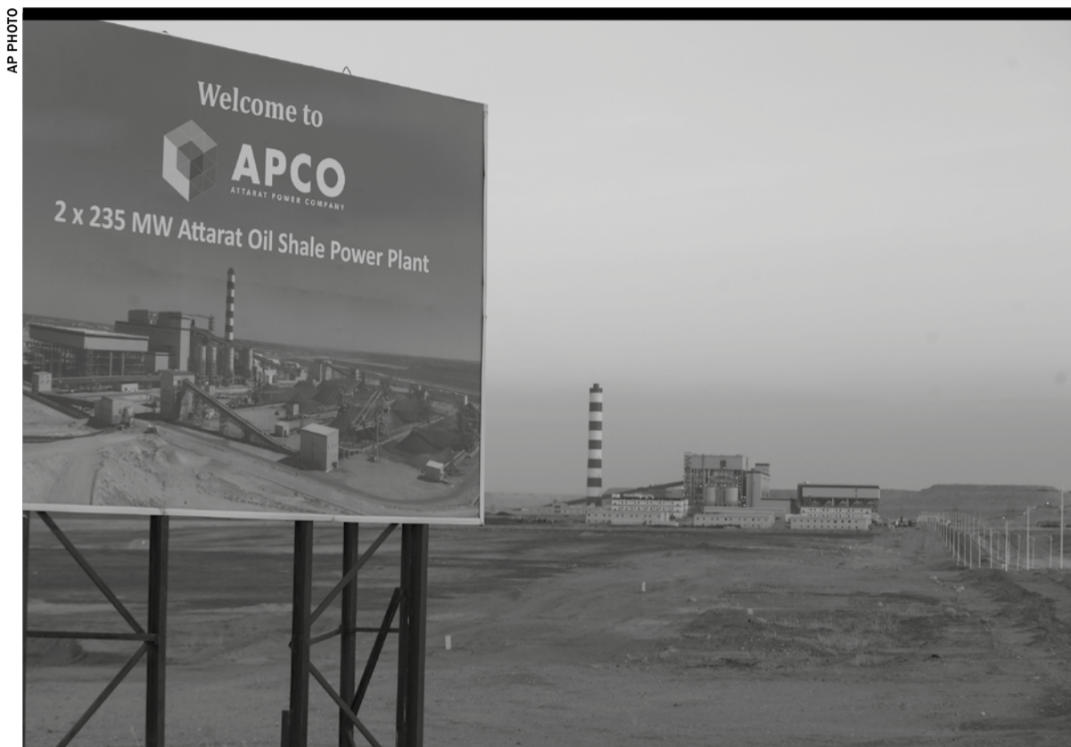
Attarat power plant is seen yesterday, some 100 kilometers south of Amman, Jordan
