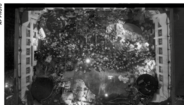
Rescuers conducting search and rescue operation at the site of a roof collapsed middle school gymnasium in Qiqihar, in Heilongjiang Province, Monday
