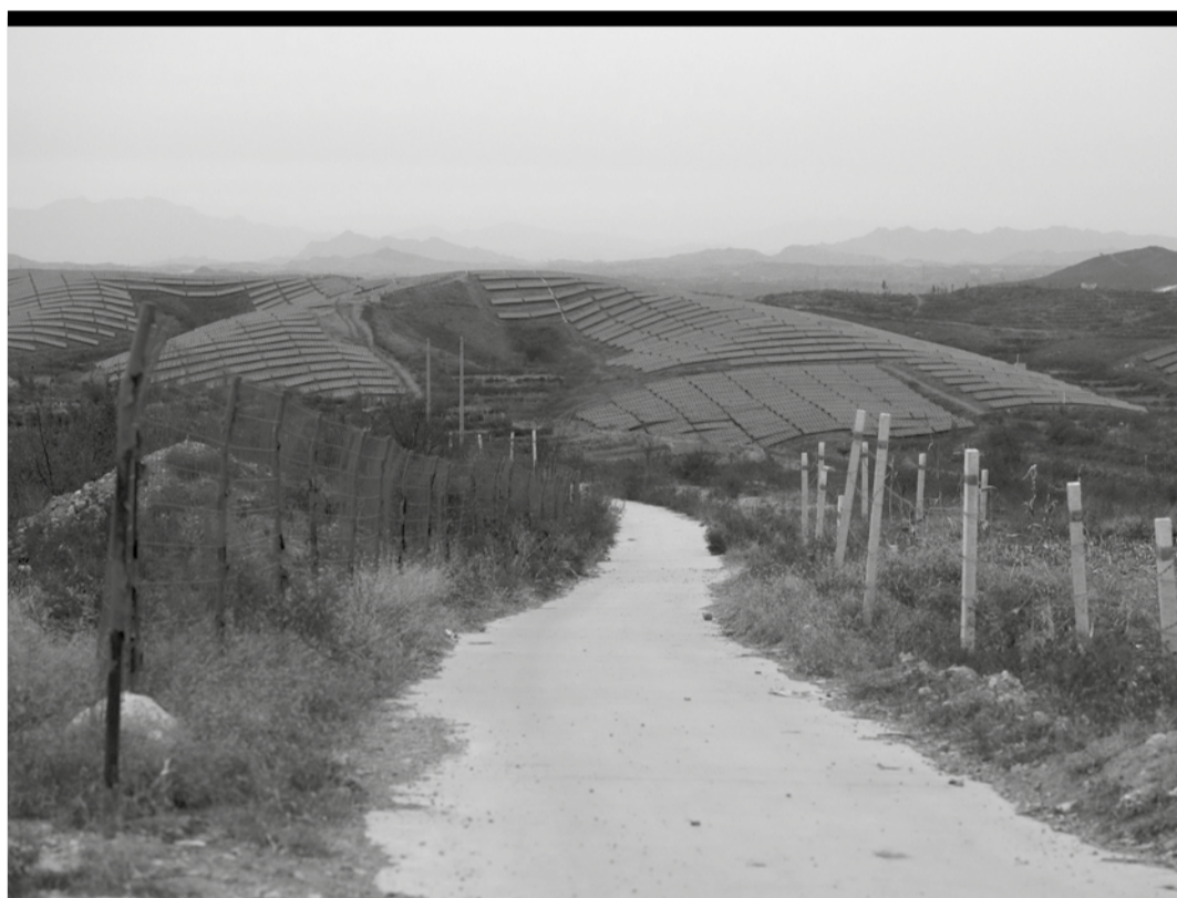
A solar farm is seen next to Donggou village near Shijiazhuang city in the northern China's Hebei province
