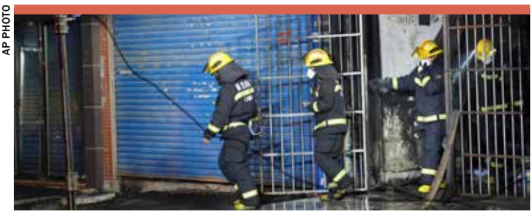
Firefighters work at the site of a building fire in Xinyu City, east China's Jiangxi Province
