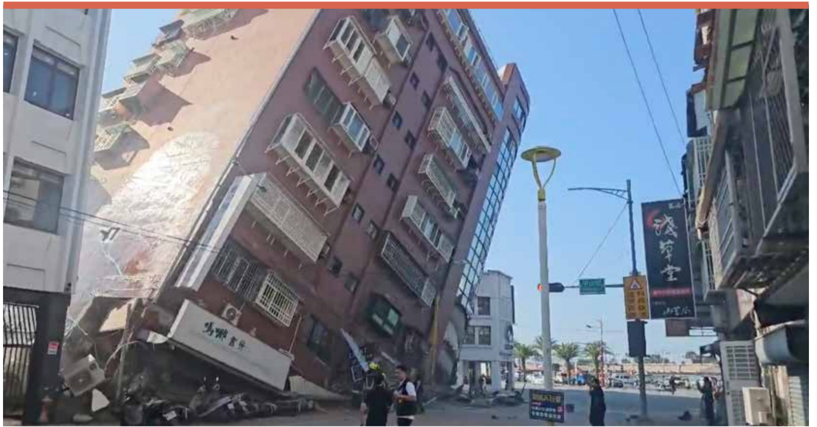
In this image taken from a video footage run by TVBS, a partially collapsed building is seen in Hualien
