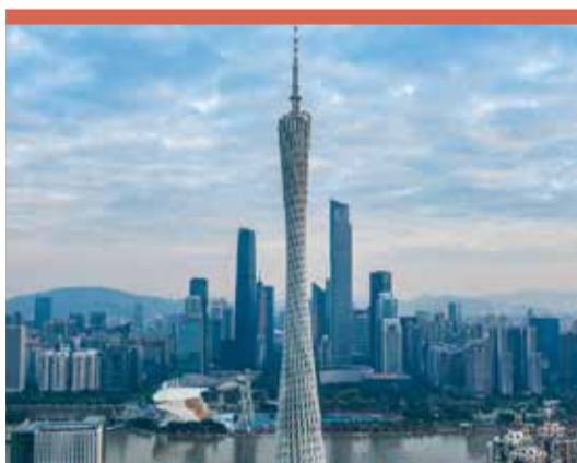
An aerial view of Canton Tower in Guangzhou
