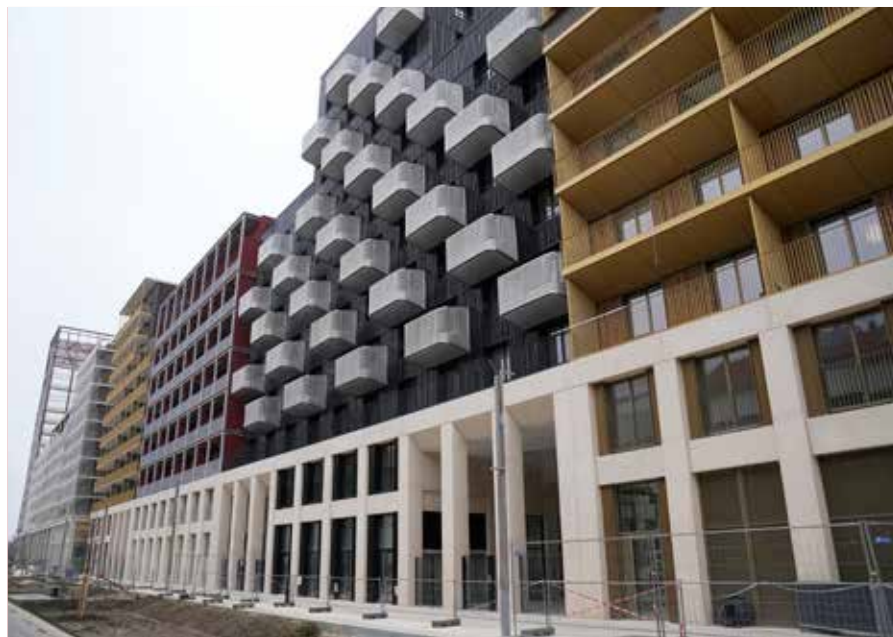
Buildings of the Olympic Village
