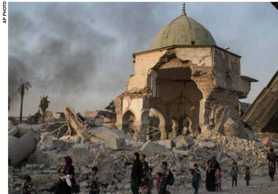
The heavily damaged al-Nuri mosque
