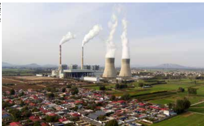
Guohua Power Station, a coal-fired power plant, operates in Dingzhou, Baoding
