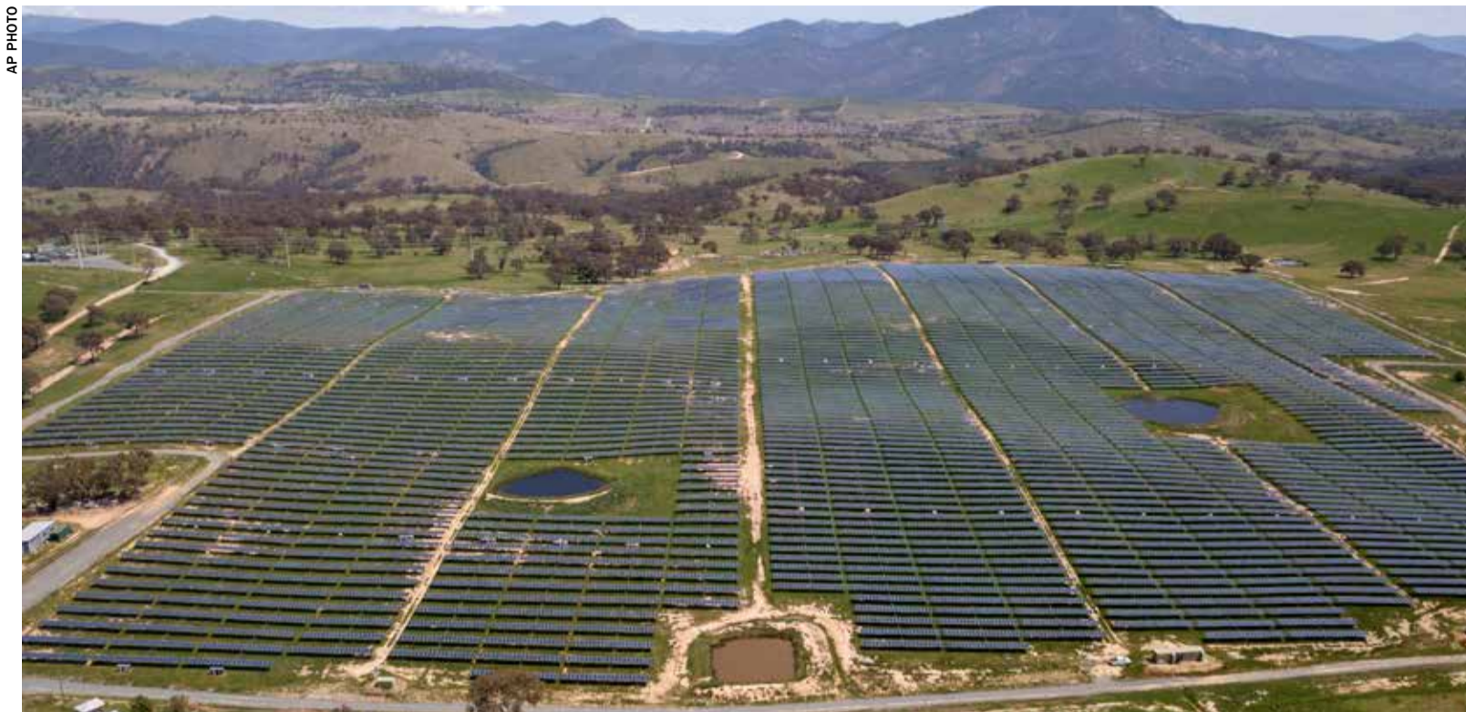
The Williamsdale Solar Farm, shown from the air and located south of Canberra
