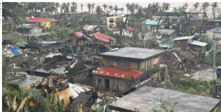
Damaged houses caused by Typhoon Man-yi in Viga, Catanduanes province, northeastern Philippines, yesterday
