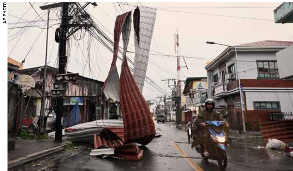
Motorists ride past a part of a roof suspended on electric wires blown by strong winds caused by Typhoon Man-yi along a street in the municipality of Baler, Aurora province
